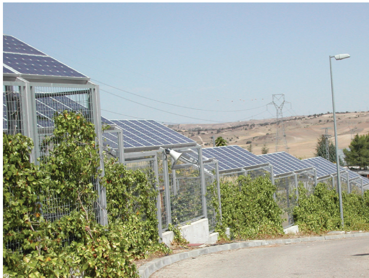
Figure 2: Power quality improvement with an energy management is tested in the experimental site of IBERINCO in San Agustin del Guadalix, Spain. PV systems may cause power quality challenges in remote areas, where the grid has not been originally designed to integrate distributed generators. (Source: IBERINCO)
